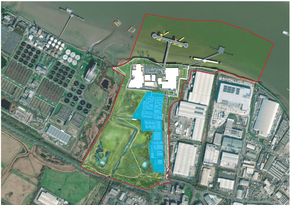
Figure 6 Carbon Capture Facility (CCF) Area
